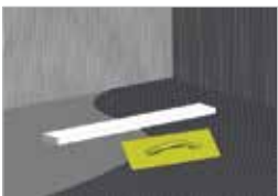
Spread the ceramic adhesive to the surface.
